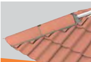
Mortar bedded security hip
